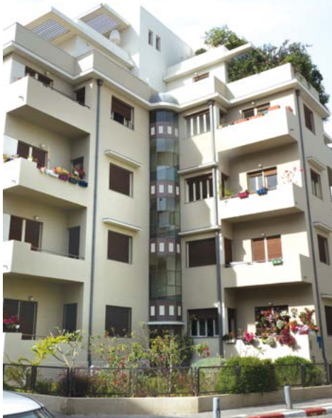
Residential building in Tel Aviv with approved two-story addition.
