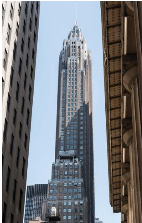
Cities Service Building, 70 Pine Street, was designed by architects Clinton & Russell, Holton & George and built 1930-31, and designated a New York City Landmark in 2011.
