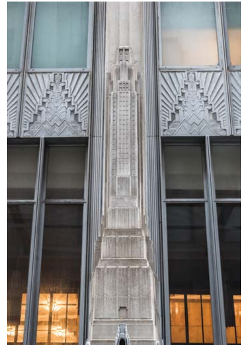
The Cities Service Building was at the time of its completion the tallest structure in lower Manhattan and the third tallest structure in the world.
