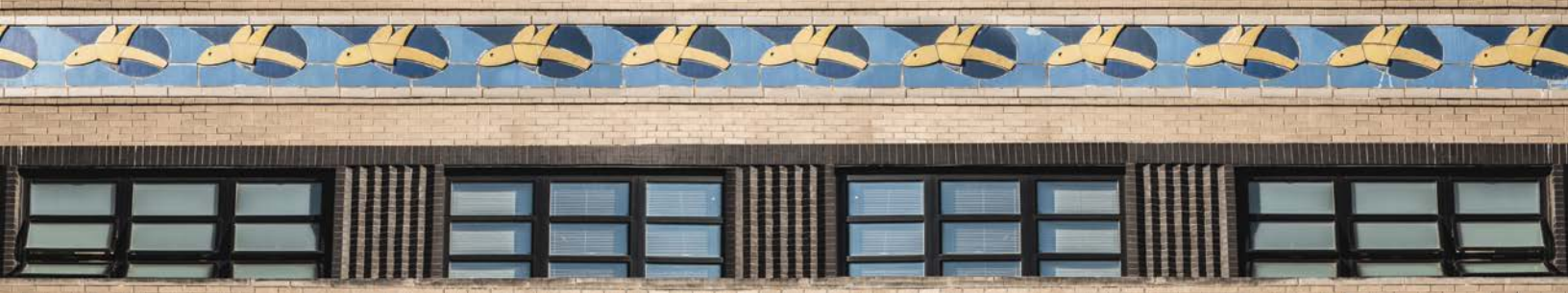
Buff and black brick around horizontally organized windows and the glazed terra-cotta band depicting flying fish, which suggests seaplanes. Photo: Lynn Farrell
