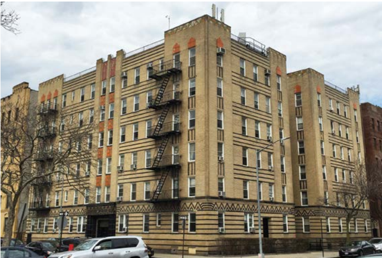
6. 711 Brightwater Court, Façade Designed in 1934 by Martyn N. Weinstein, this perfectly maintained building boasts vibrant terra-cotta spandrels, clean-lined banding created with alternating black and beige brick, a single band of chevron patterning, as well as a breathtaking black and gold terra-cotta entrance. The lobby has been very well maintained.
