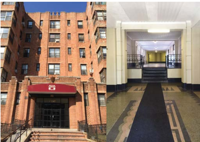
1. 3100 Ocean Parkway, Façade and Lobby The beauty of this Art Deco residential building from 1932 is attributable primarily to the brick patterning of the entrance and spandrels. The central design in the lobby's terrazzo floor and the fluting on the ceiling guide visitors through public spaces.
