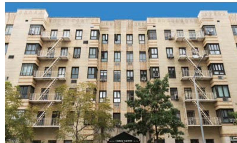
6. 255 West 23rd Street The 1937 Chelsea Gardens is a rare garden apartment building in Manhattan. The main entrance features an ornate surround and apartments overlook a central garden.
