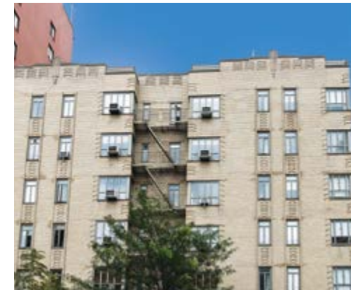
4. 155 and 165 West 20th Street On the northeast corner of Seventh Avenue, the Warren Apartments feature ornamental brickwork, corner windows, and handsome lobbies with brightly colored terrazzo floors. It was designed in 1938 by Horace Ginsbern, architect of the "Fish Building" on the Bronx's Grand Concourse.
