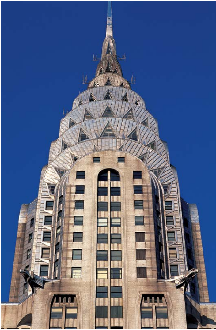
LEFT: Nirosta crown of the Chrysler Building with its seven concentric ribbed steel arches set with triangular windows. Photo: Richard Berenholtz
