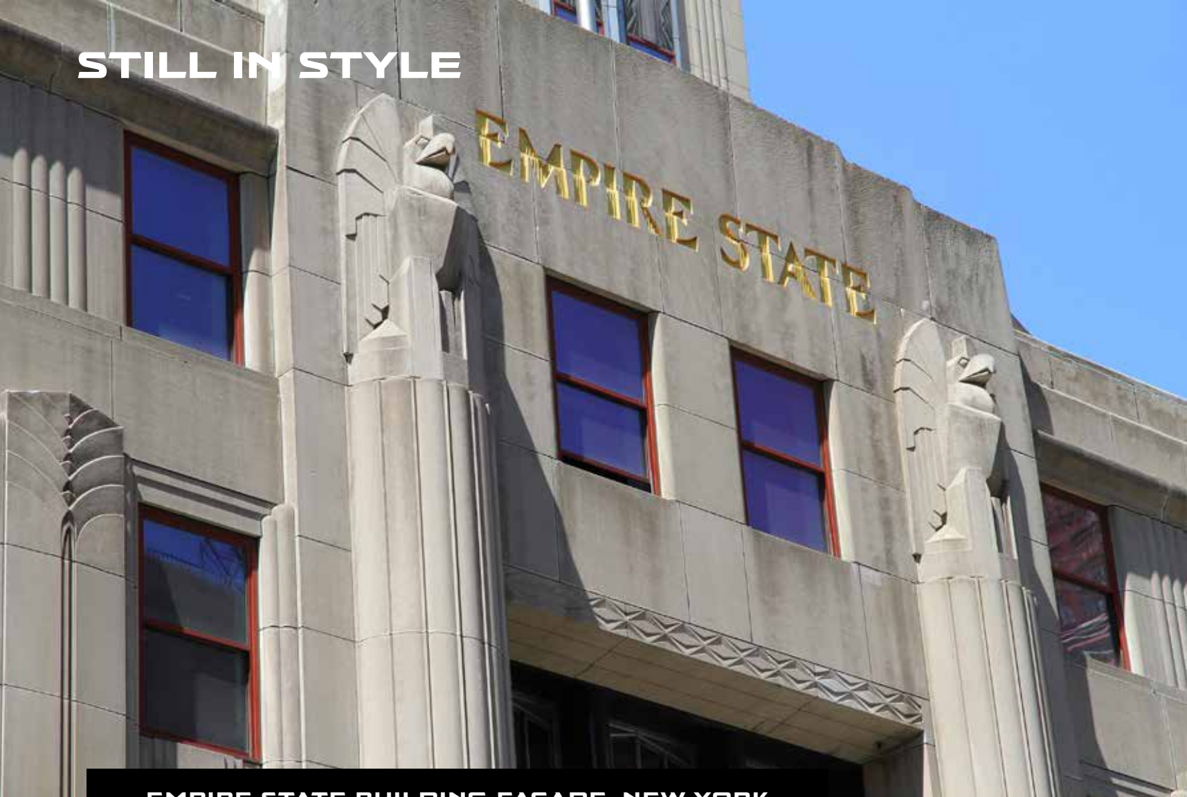
EMPIRE STATE BUILDING FAÇADE, NEW YORK
