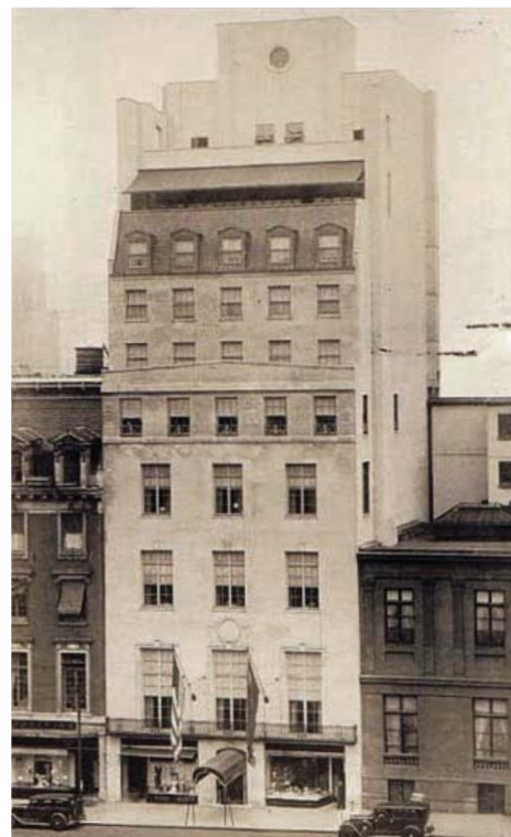
TOP TO BOTTOM: Construction photo of “The Panhellenic” featured on a postcard postmarked 1929.
